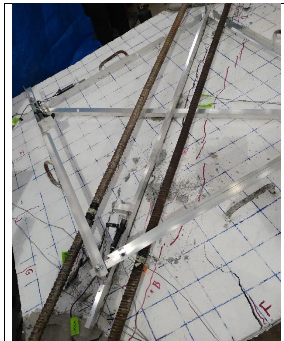
Figure 3.12 : The noticeable cracks of the voided slab.
