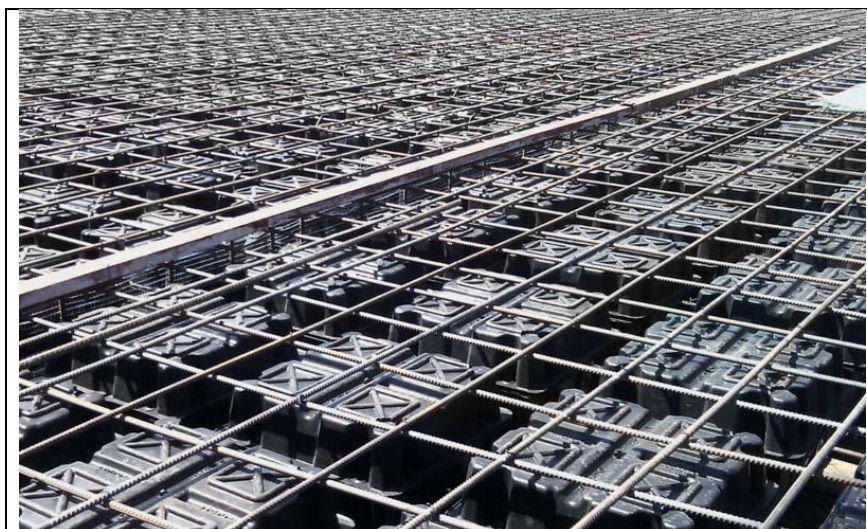
Figure 1.7 : The circular or bubble deck
