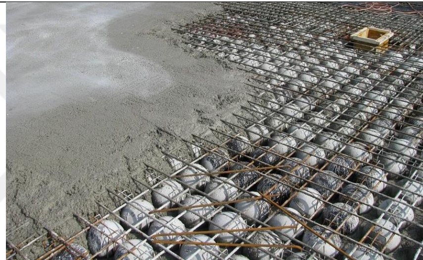
Figure 1.7 : The circular or bubble deck
