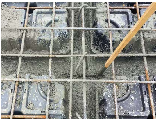
Sample 4: Plasticization of the concrete and second stage of casting
