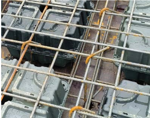
Sample 3: Connecting to the steel below and controlling concrete casting through the central cone
