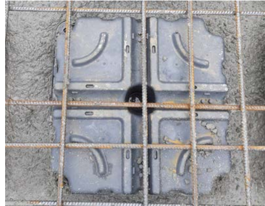
Sample 3: Connecting to the steel below and controlling concrete casting through the central cone
