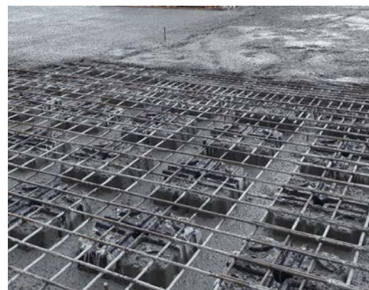
Sample 4: Plasticization of the concrete and second stage of casting
